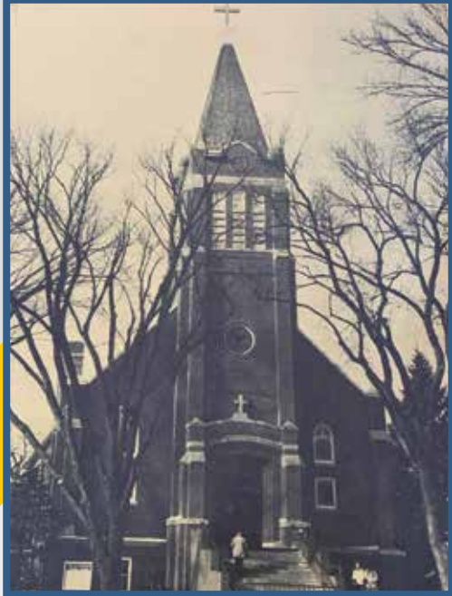
The old Our Lady of Victory Church suffered a major fire just before the start of Holy Week services in 1961. The church was repaired and again became operational in early 1962.
